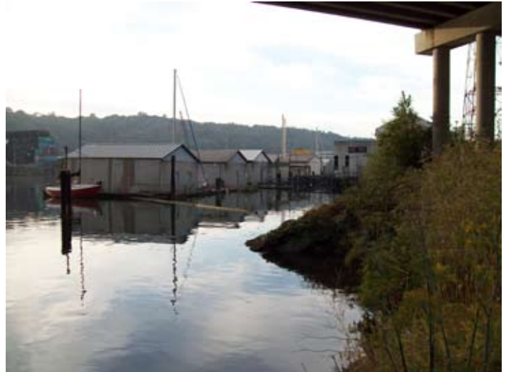
Existing recreational boat moorage, east bank line, First Avenue South Bridge (River Mile 2.0)
