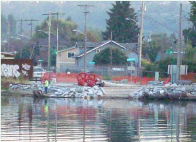
Existing restoration at Portland Street
