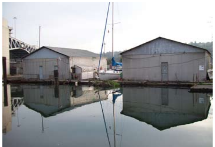
First Avenue South Bridge, illustrating potential restoration area between top-of-bank and floating moorage (River Mile 2.0)
