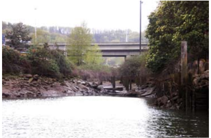
Existing side channel, intertidal pocket, west shoreline, (River Mile 2.4). This area is located between projects 11 and 13. It illustrates a potential restoration opportunity involving private property owners and the Port.
