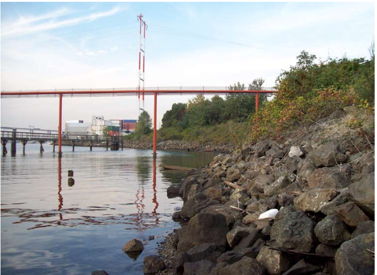
Terminal 108, riprap bank line, illustrating potential marsh and riparian vegetation pocket restoration site (River Mile 0.5)
