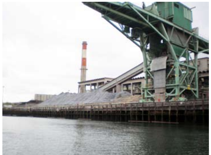
Large scale water-dependent, marine industrial pier facility (River Mile 1.0)
