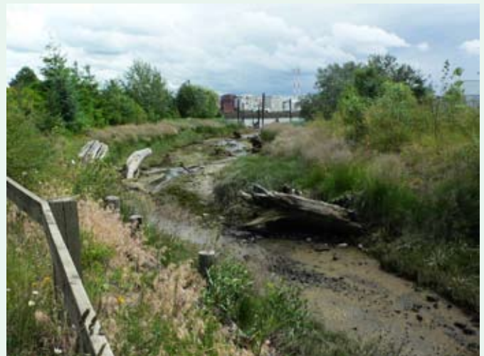
Existing restoration at terminal 105
