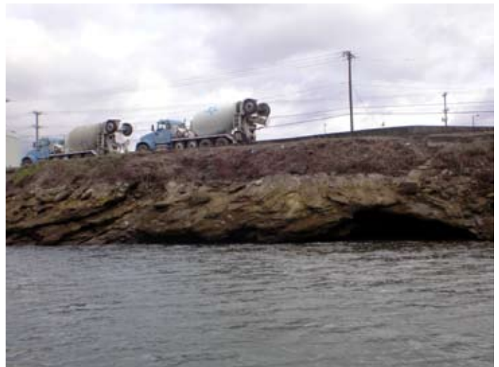
Artificially hardened and eroded bank at east side slip (River Mile 1.8)
