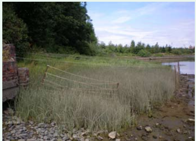
Existing restoration at terminal 107
