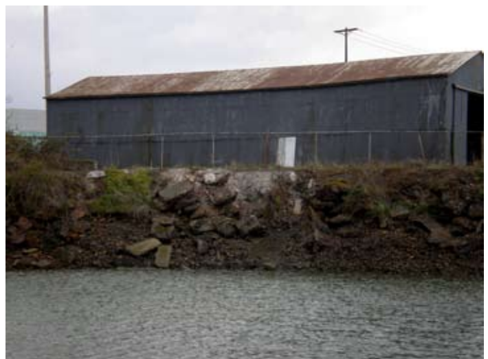
Illustrating rubble, industrial fill shoreline, east bank, (River Mile 3.8)
