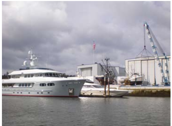
Existing marine industrial use, west shoreline (River Mile 4.4)
