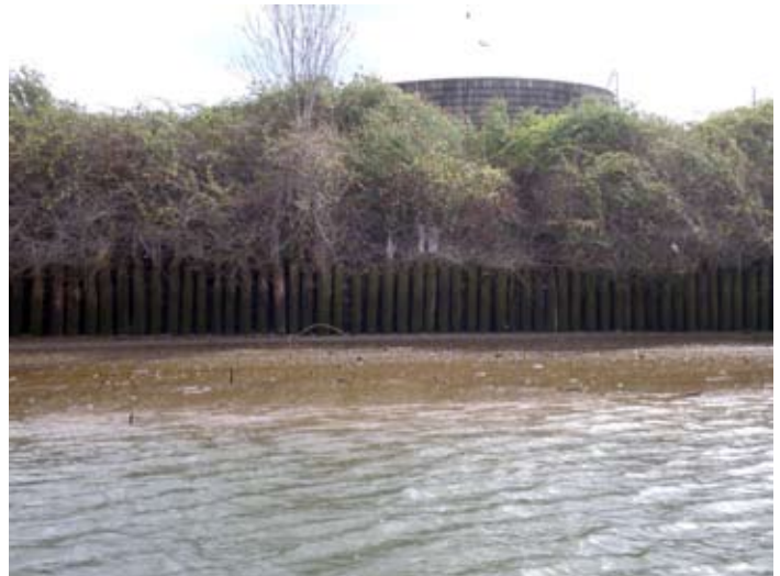
Existing creosote timber bulkhead, east bank line (River Mile 3.8)
